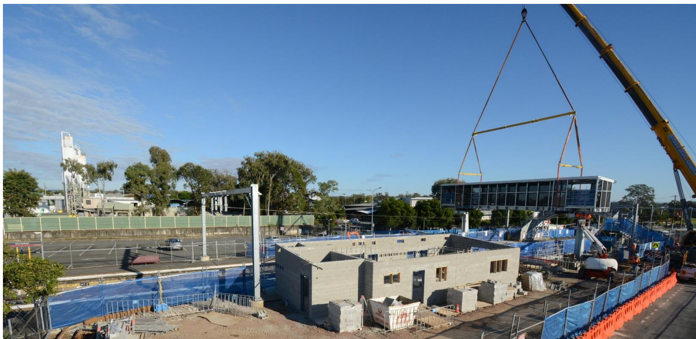
Installing new footbridge during scheduled track closure, early June.
